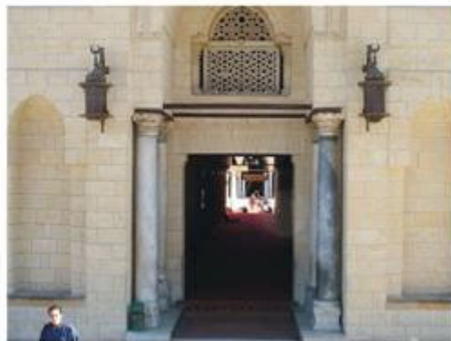
Amr Ibn- Al- Ass Mosque Wall (A-site)
