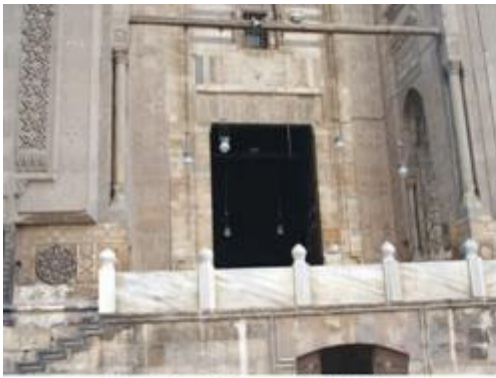
Sultan Hassan Mosque Wall (H-site)
